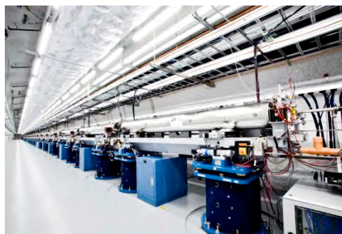
Figure 17: view of the 100 m long undulator of the Linac Coherent Light Source.
