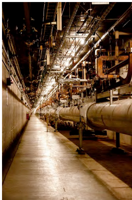
Figure 4: A view inside the two-mile SLAC accelerator tunnel showing the linac mounted above the alignment light pipe.
