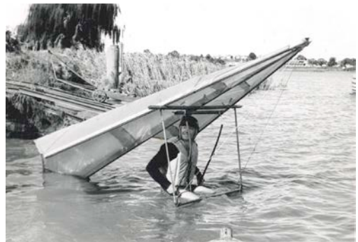
Figure 5. Half-size model waiting for a test run in 1963. Pilot John Dickenson.
