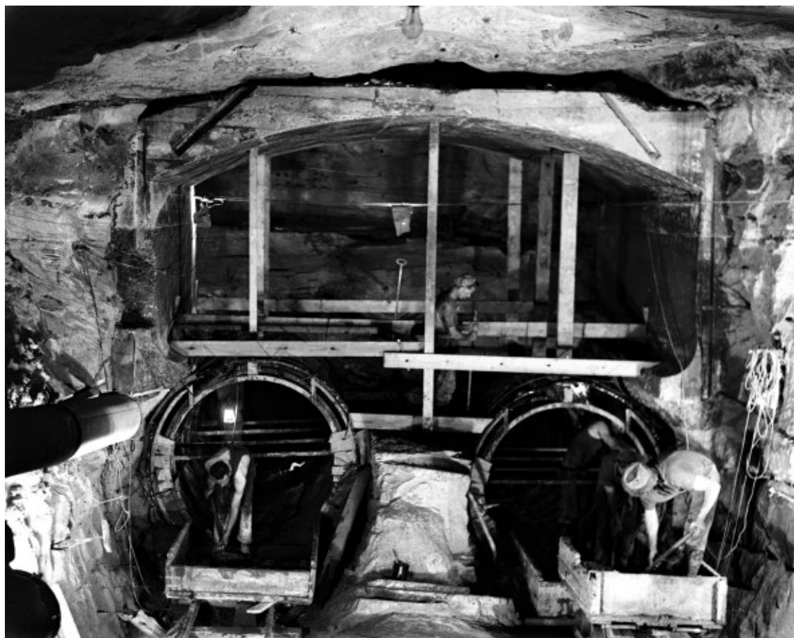
Figure 6: Construction of the Southern and Western Ocean Outfall System (c1915).
