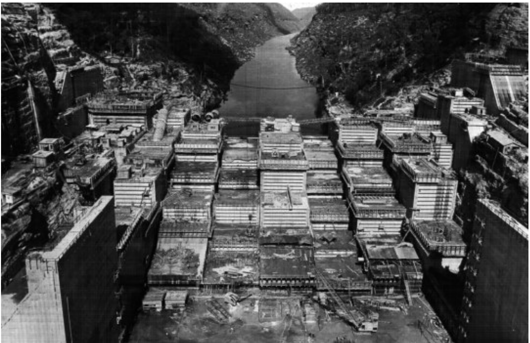
Figure 10: Warragamba Dam main wall construction.
