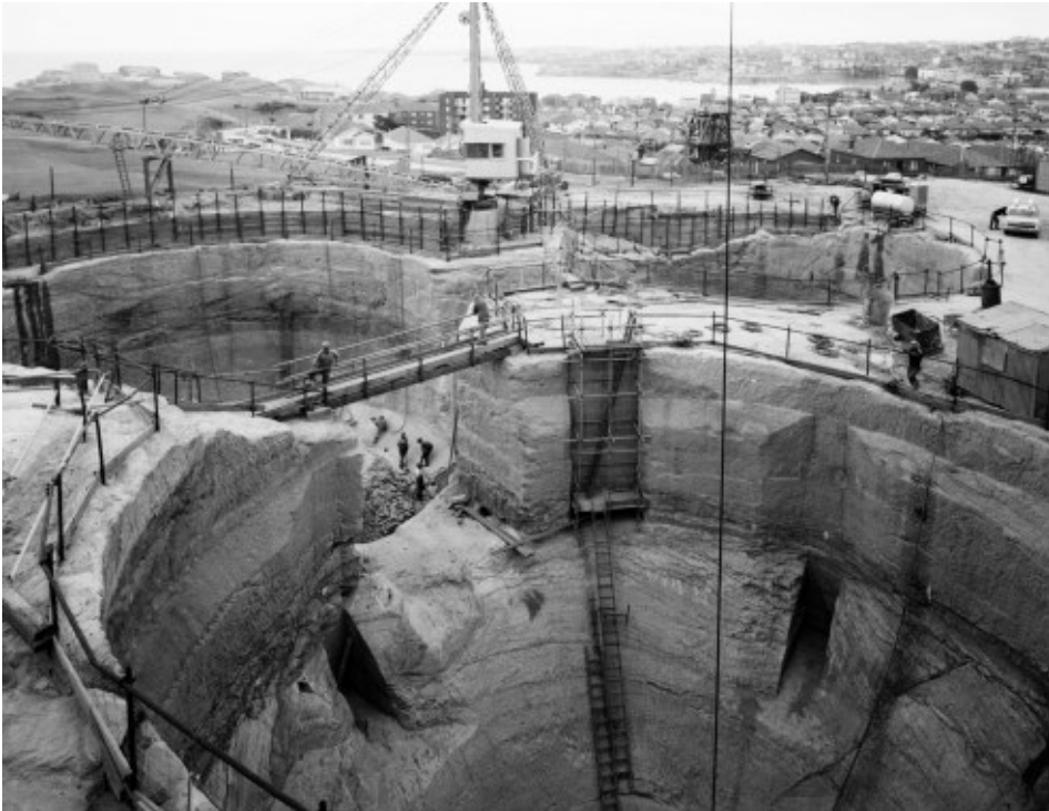
Figure 12: Bondi Sewerage Treatment Works under construction in 1984.
