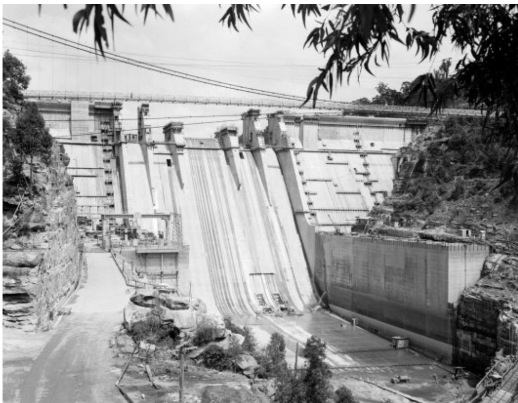
Figure 11: Warragamba Dam nears completion.
