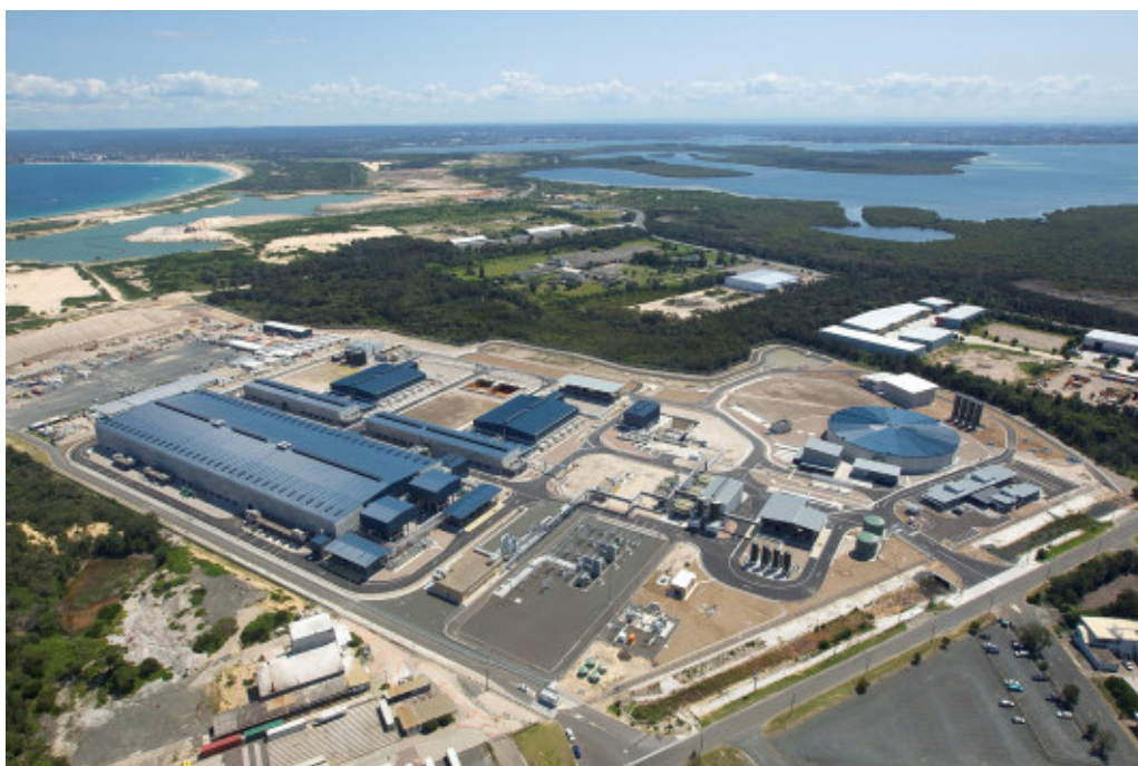
Figure 13: Desalination plant, Kurnell, 2008.
