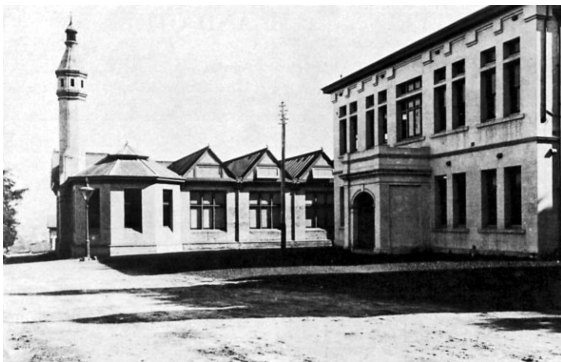
Figure 3. School of Mines/Geology building (right), former Engineering Building (left).
