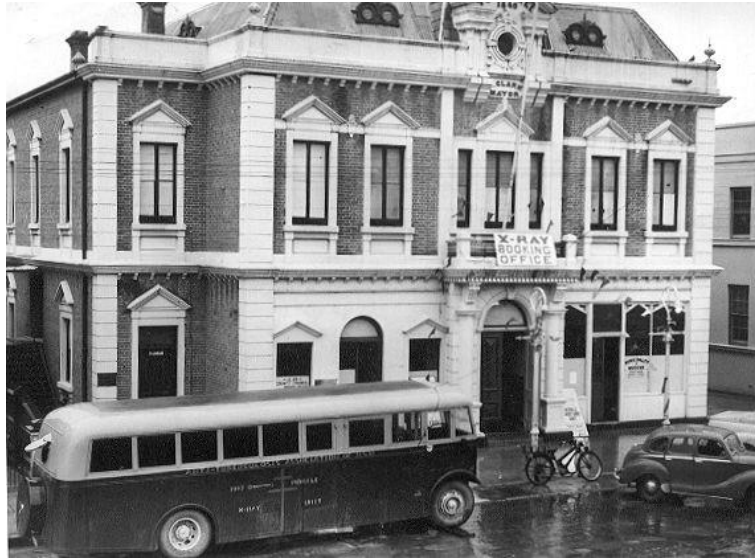
A Mobile Xray Bus at Mudgee. The original mobile X-ray units travelled in a converted Sydney bus, which included space for a photographic darkroom and a radiologist's consulting room. The large X-ray machines of this era had to be unloaded from the bus and set up in a building, usually the local Town Hall.
