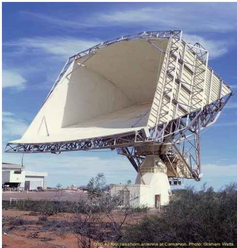
Figure 7: The original Cassegrain horn antenna at the first Australian INTELSAT satellite Earth station in Carnarvon, Western Australia.
