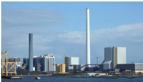
Diagram 10: Kalundborg Power Station in Denmark, CC0
