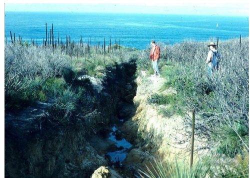
Figure 1: A previously in-filled and subsequently deeply gullied section of the Coast Walk, 1991.
