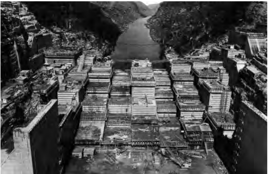
Figure 10: Warragamba Dam main wall construction.
