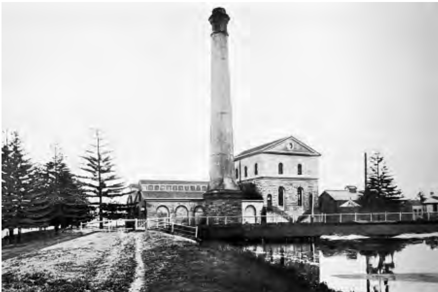
Figure 4: Botany pumping station (c1870?).
