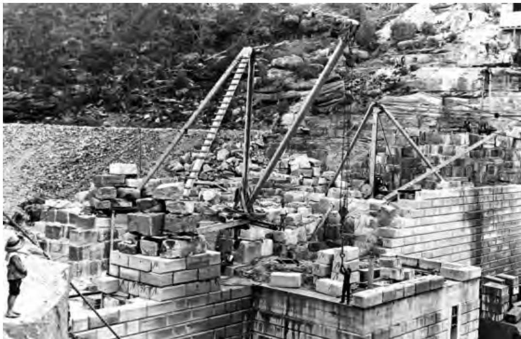
Figure 7: Cataract Dam under construction (c1905).
