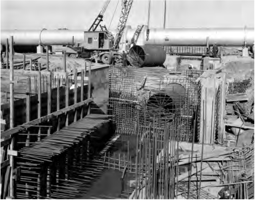
Figure 9: Warragamba Dam under construction. The photo shows No. 2 Cross Connection. Looking south at the cross pipe showing Mk. 26 under the crane. Partly constructed 84 inch valve chamber in foreground.
