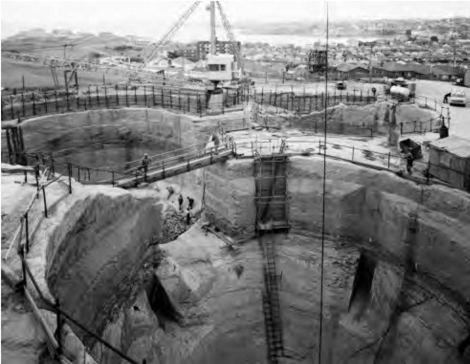
Figure 12: Bondi Sewerage Treatment Works under construction in 1984.
