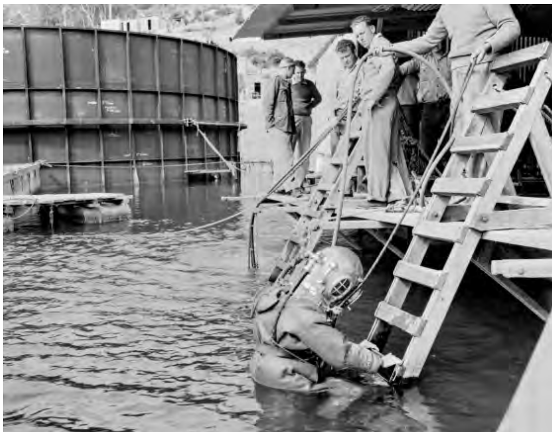
Figure 8: A diver entering the water at the Avon coffer dam.
