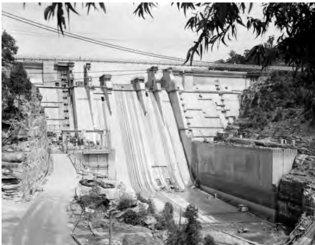
Figure 11: Warragamba Dam nears completion.
