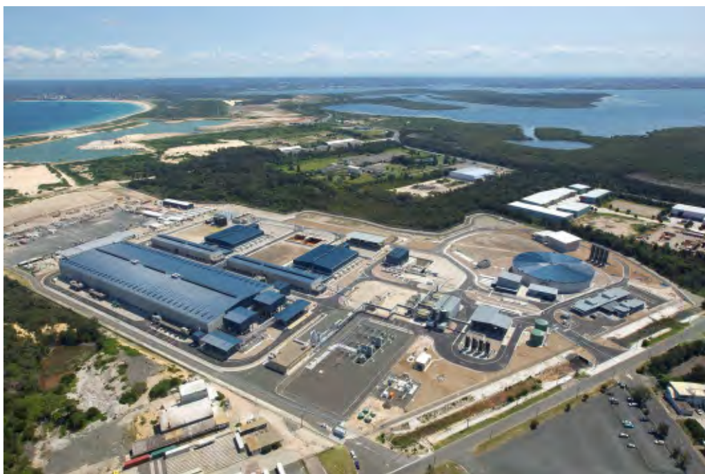
Figure 13: Desalination plant, Kurnell, 2008.
